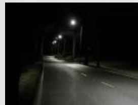
30 Watt LED-lamps replacing 125 Watt HQL-lamps ( federal road in Vogtland)
